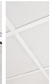
Suspended Ceiling Grid
